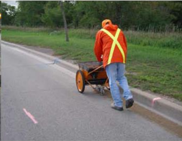
(ii) Applying Test Material Along The Curb
