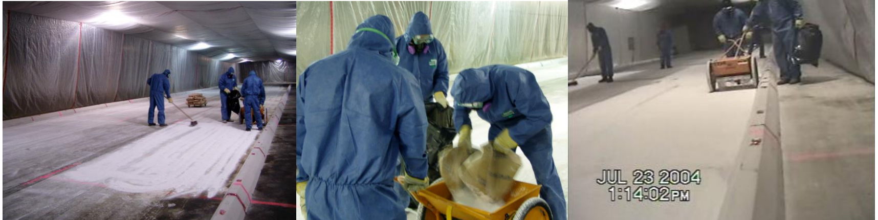
Figure7: Application of Test Material
