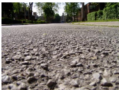
Figure 1c Severe Raveling
