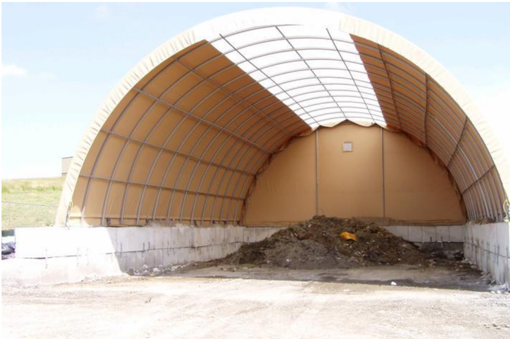
Figure 9: Enclosed Street Sweeping Pit
