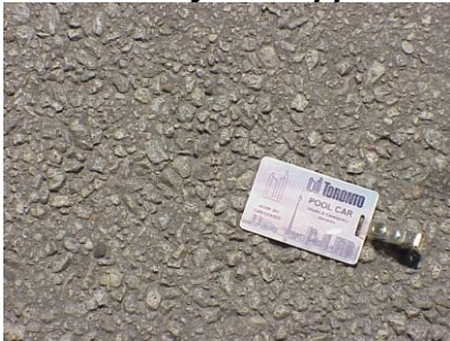
Figure 1a Slight Raveling
