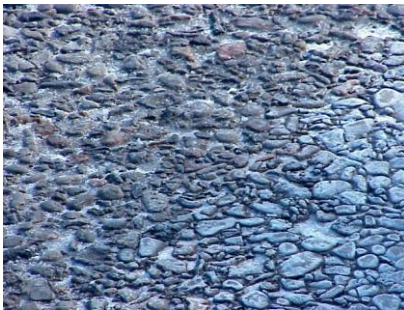
Figure 1b Moderate Raveling
