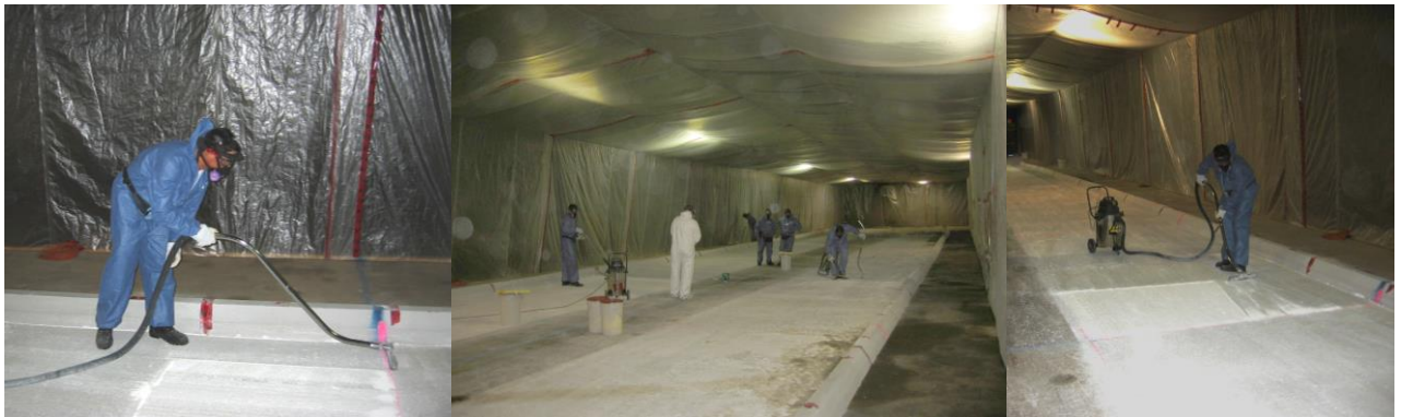
Figure 12: Vacuuming of Residue Material
